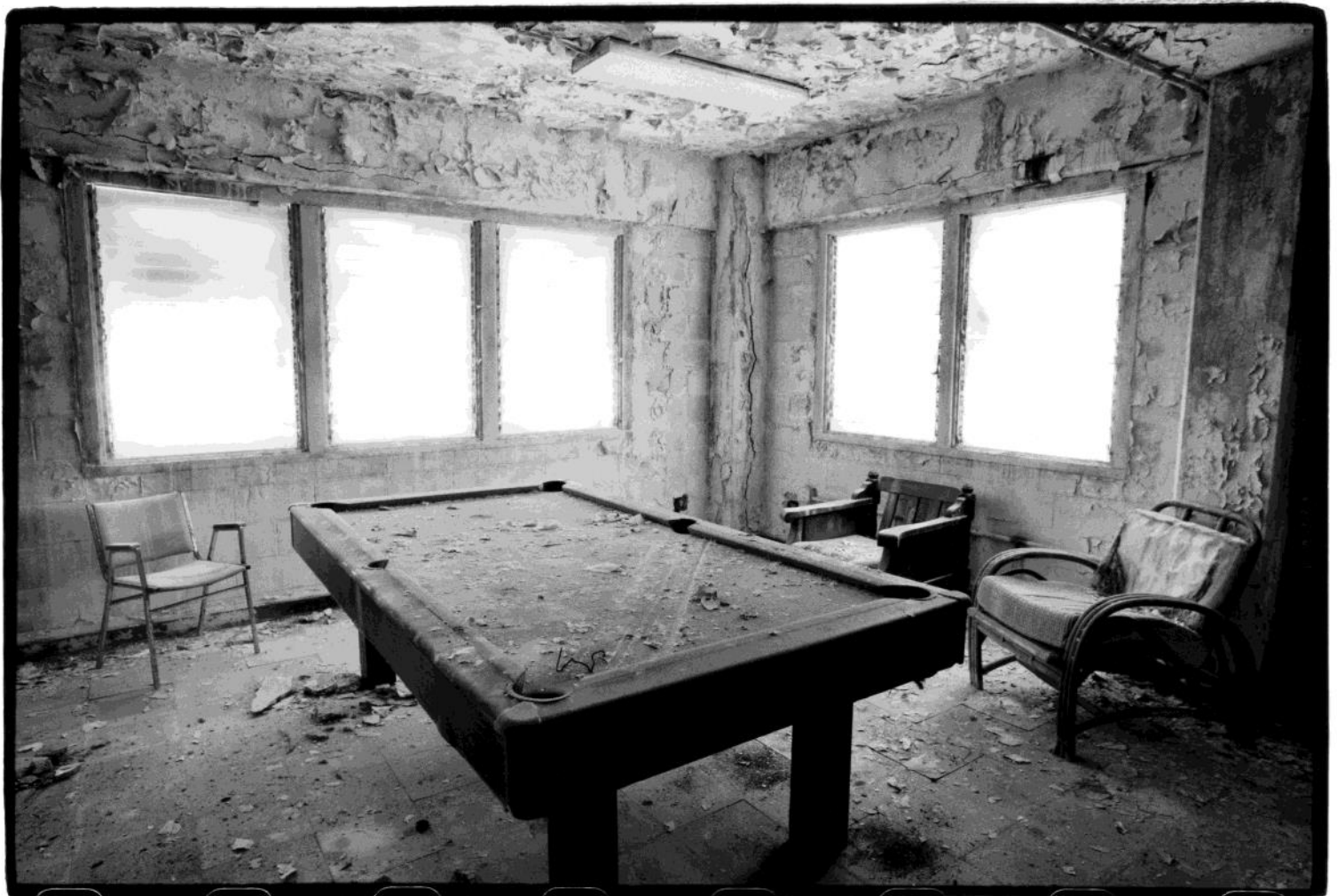
Peeling layers of paint and crumbling concrete now adorn the walls of the recreation room inside the Delta Barracks.
