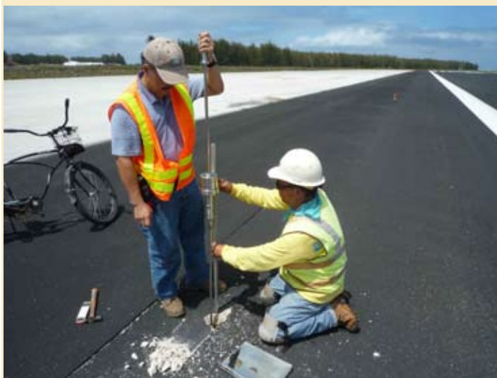
Engineers checking soil compaction under trench.
